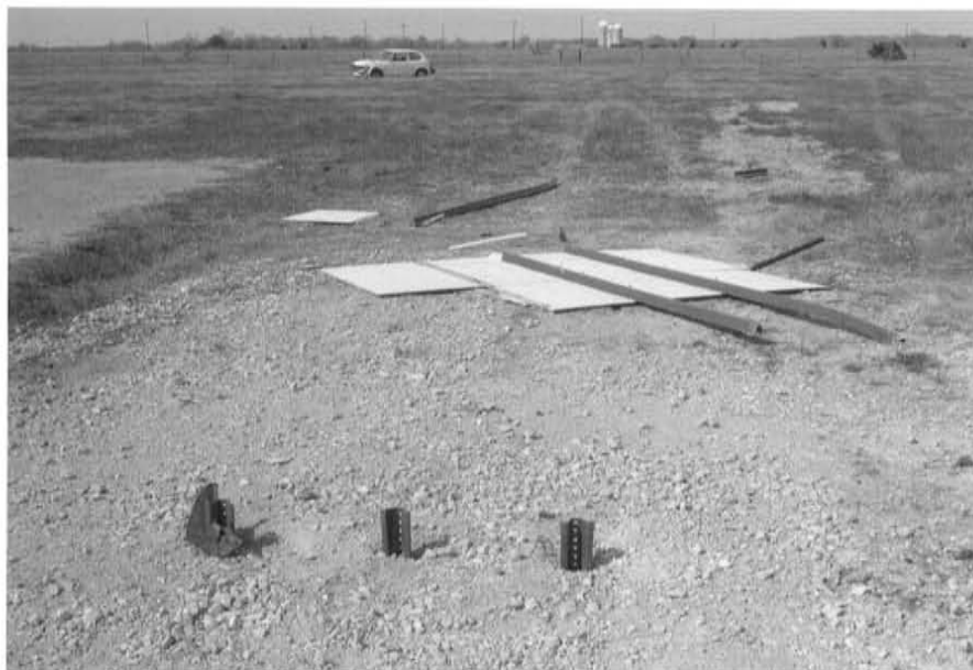
FIGURE 7.9. SIGN INSTALLATION FOLLOWING TEST 7024-25.
