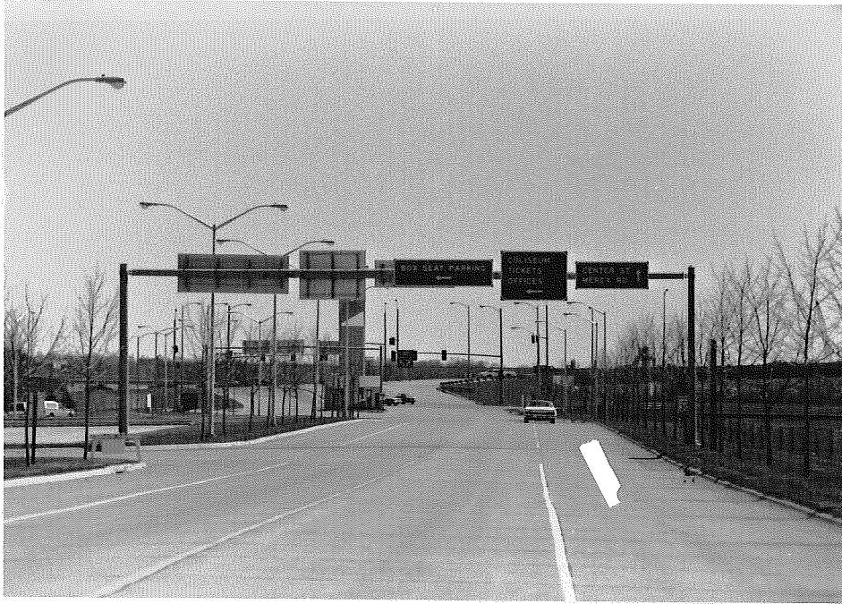
Fig. 1.1 Typical Monotube Sign-Support Structure (Courtesy of Valmont Industries, Inc., Valley, Nebraska)
