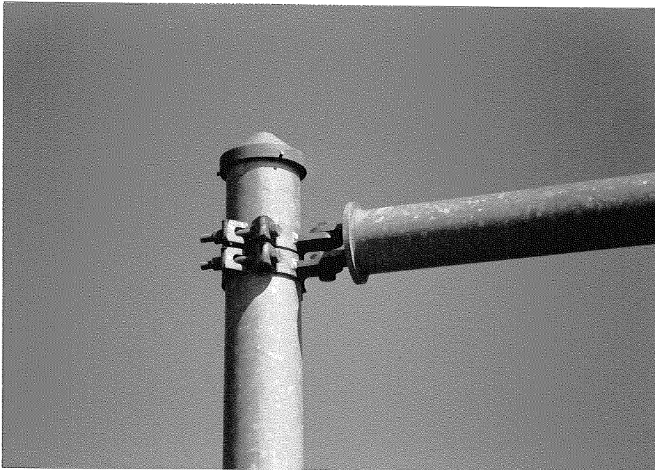
Fig. 1.2 Beam to Column Connection for a Sign-Support Structure (Courtesy of Valmont Industries, Inc., Valley, Nebraska)
