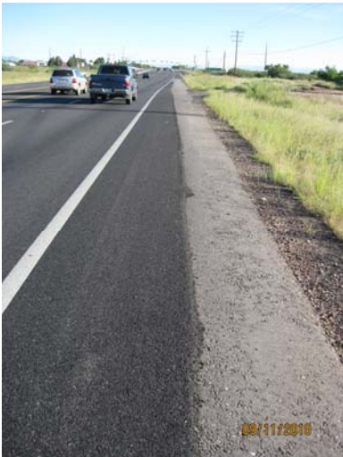
Example of an irregular shoulder on SR 92 that can cause a hazard to bicycle riders Photo Source: Thomas Armstrong
