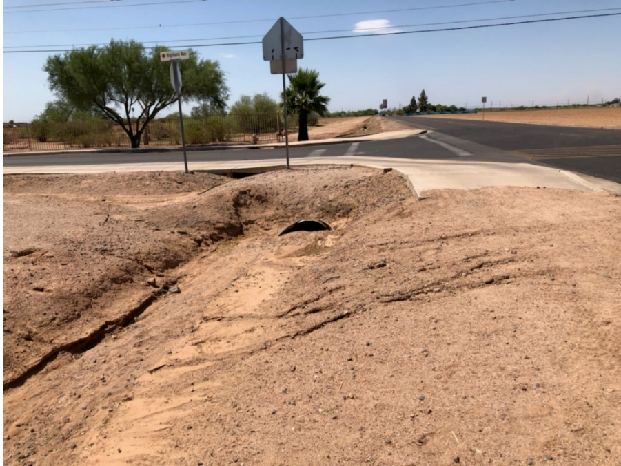
Figure 1. Cross culvert in poor condition due to sediment loading.
