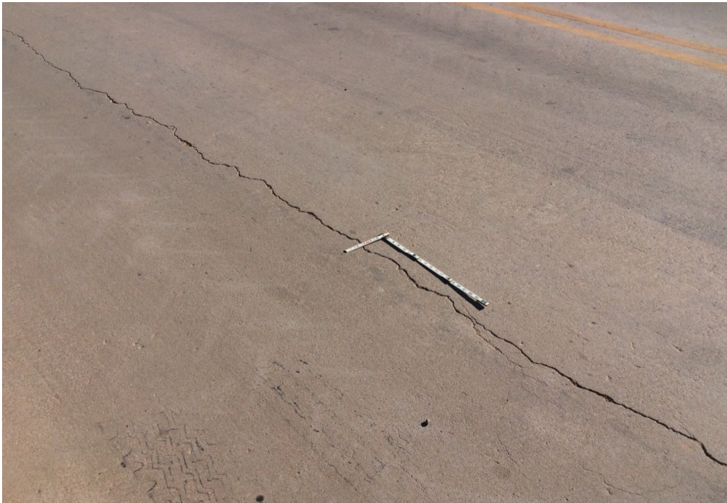
Full length longitudinal cracks in bridge deck
