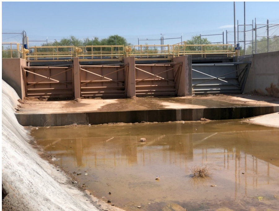
Figure 5. Arizona Canal overflow gates
