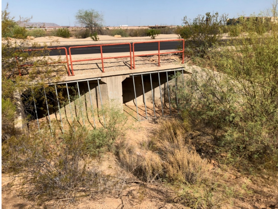
Figure 3. Dual cell RCBCs (7-ft x 8-ft) along Dobson Rd.
