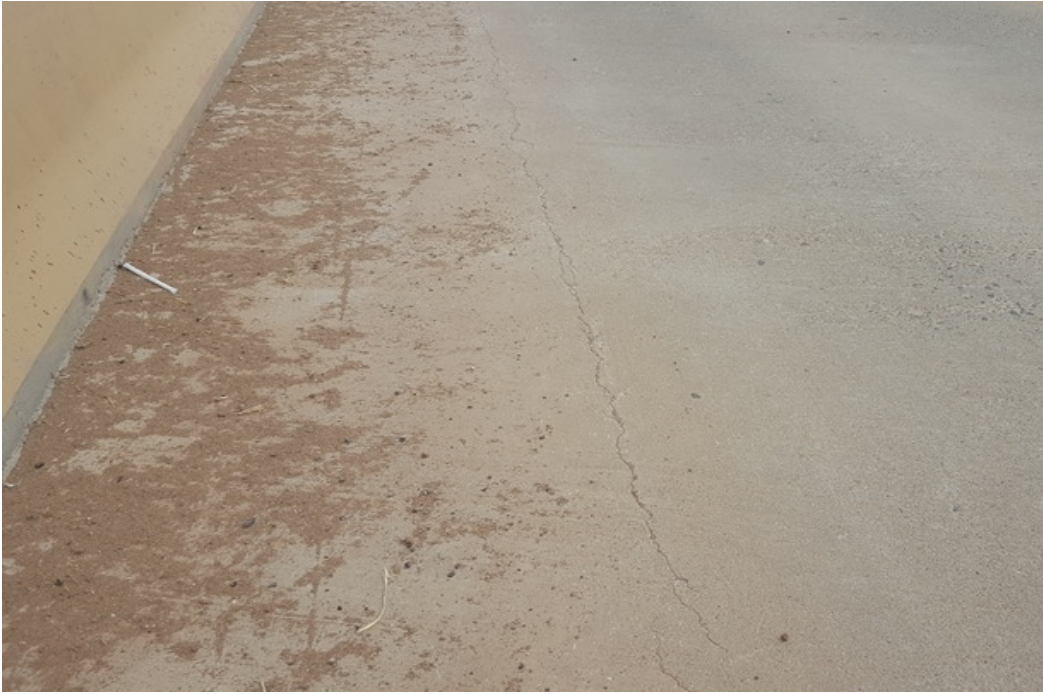
Full length longitudinal cracks in bridge deck
