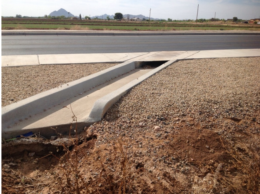
Figure 2. Curb inlet and concrete scupper along Center Street.
