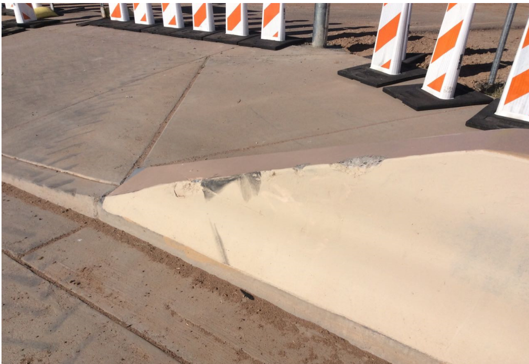
South West corner, impact damage to concrete barrier
