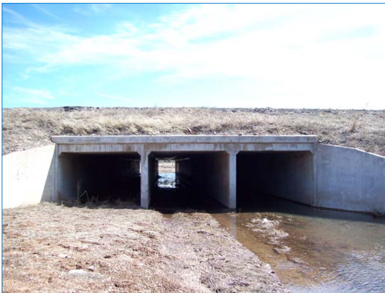
Culvert under I-17, adjacent to Tovar Trail. The left culvert could potentially be used as a pedestrian crossing to the east side of I-17.
