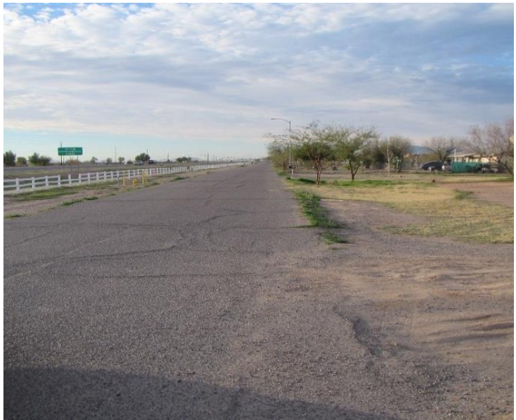
Paving on Antone Avenue showing raveling of the pavement edges and transverse cracking. This road is planned to be reconstructed.
