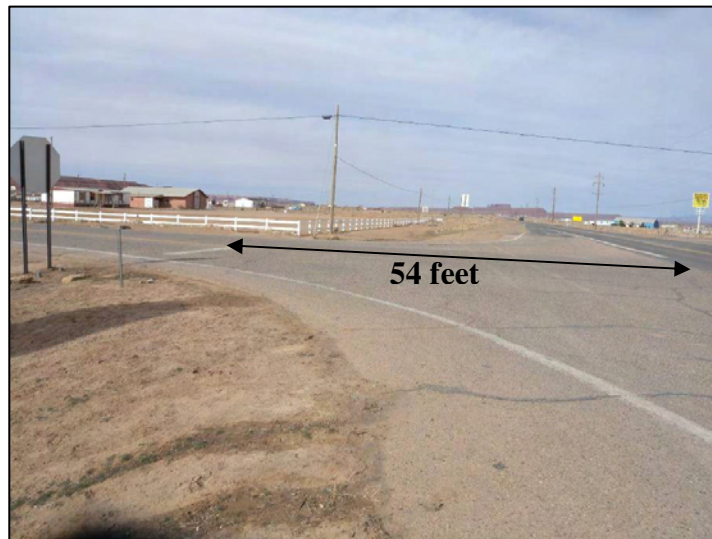
Figure 16: Stop Bar at N59 is Located 54 Feet From the Through Lane
