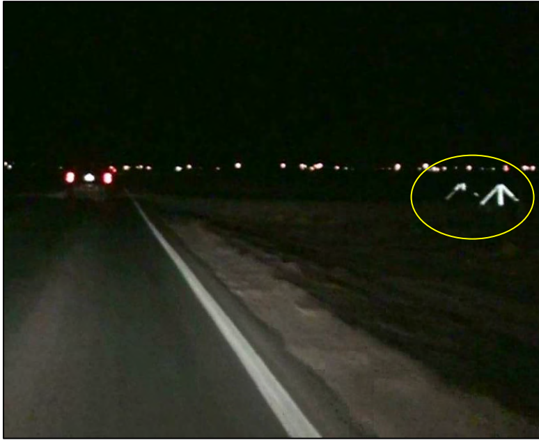
Figure 9: Delineated Cattle Guards Can Help Drivers Locate Intersections
