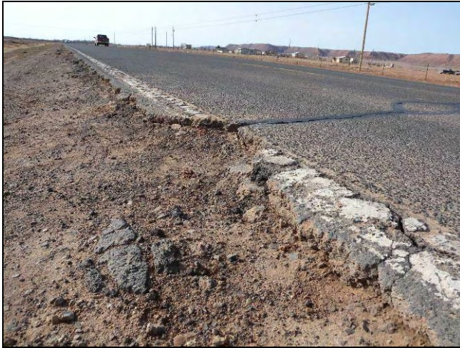
Figure 2: Lack of Paved Shoulder and Pavement Edge Deterioration
