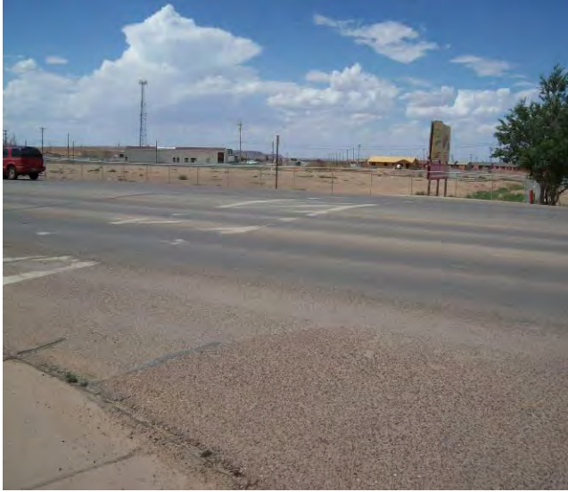
Pedestrian crosswalk in Chinle (N7) with striping that has been worn away.
