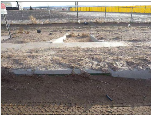
Figure 17: Clogged Drain Under Sidewalk and Sidewalk Covered with Debris in Chinle
