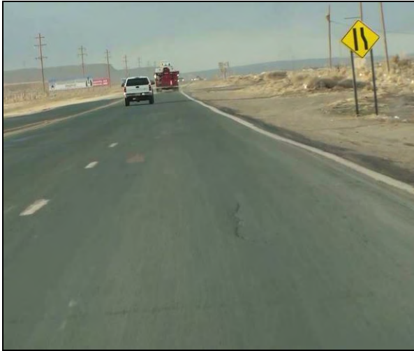
Figure 11: Right Lane Ends Sign at MP 448.27 Appears to be Too Close to Taper
