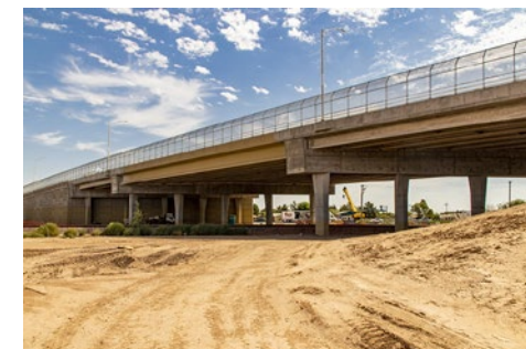
When this photo was taken in July, SR 347 improvements were about 80% complete. Today, ADOT is adding finishing touches.
