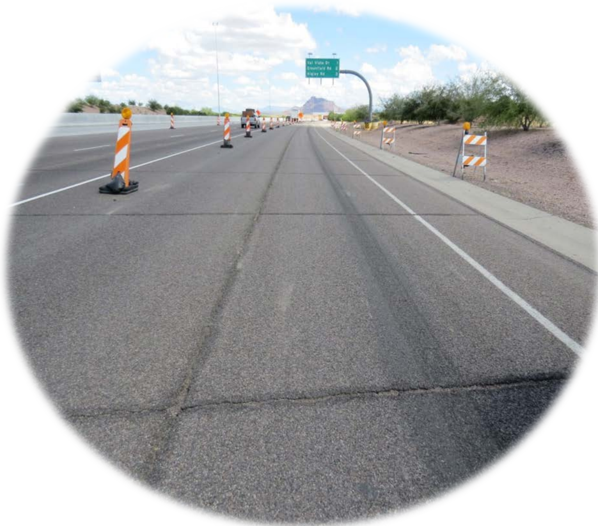
Cracking (Unacceptable)
