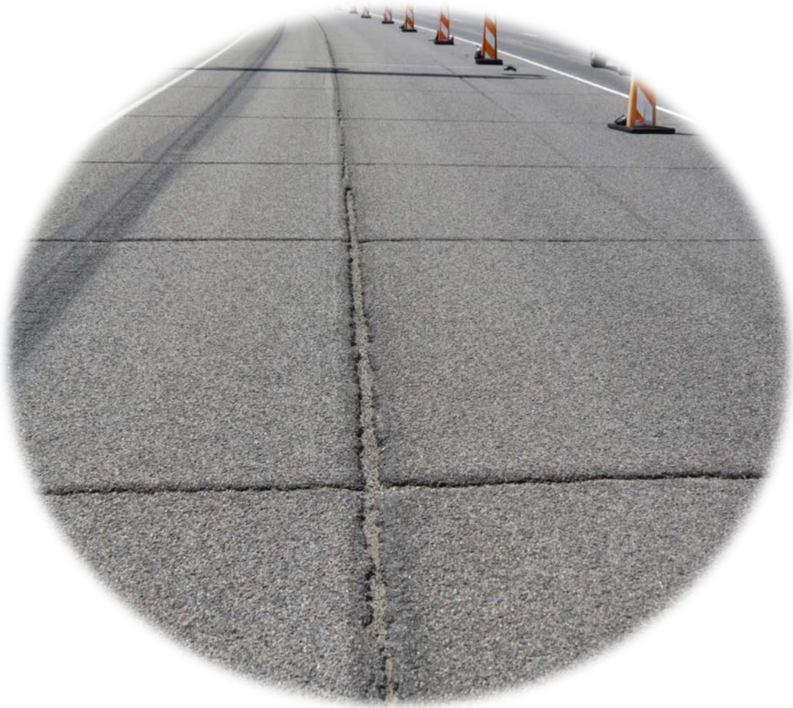
Cracking (Unacceptable)
