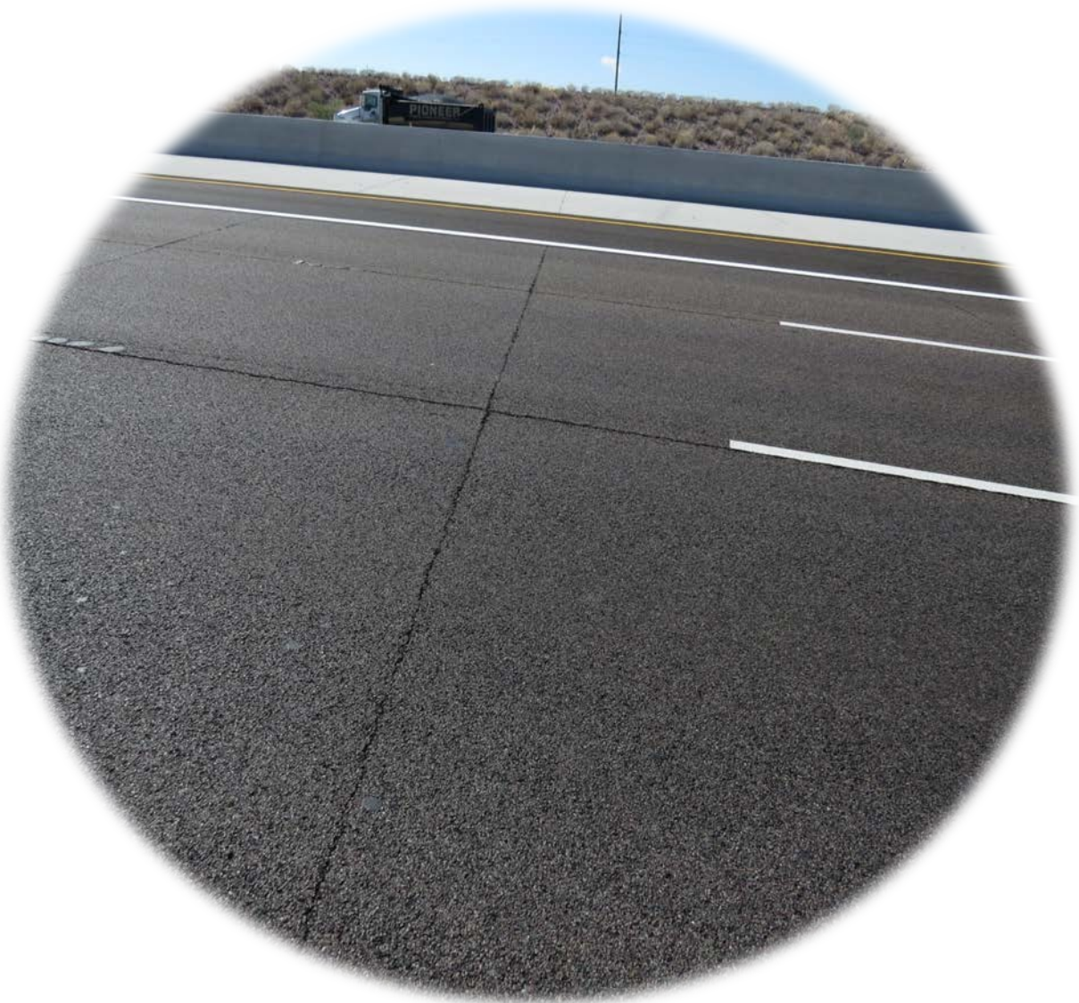
Cracking (Acceptable)
