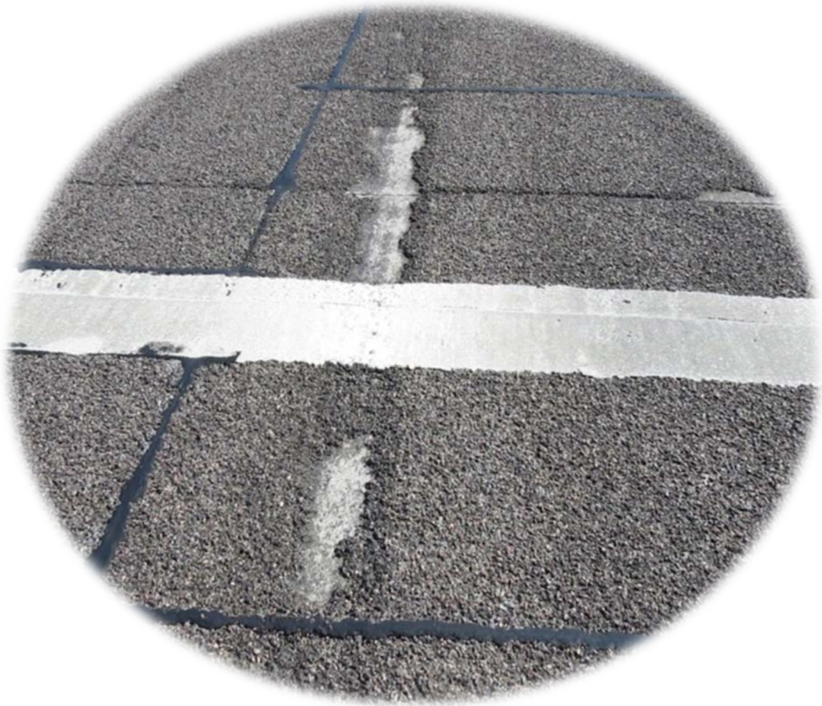
Delamination (Unacceptable)
