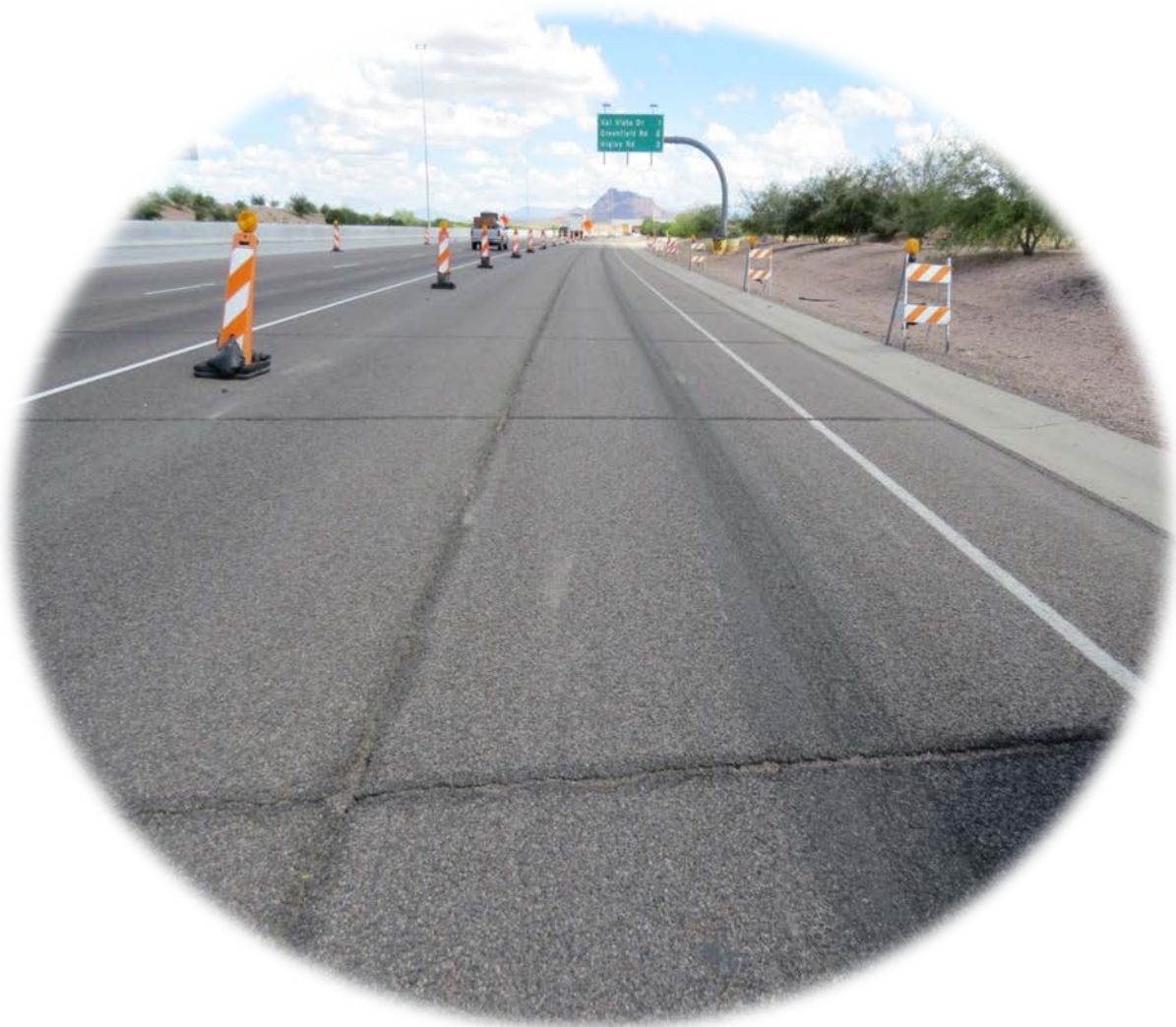
Cracking (Unacceptable)
