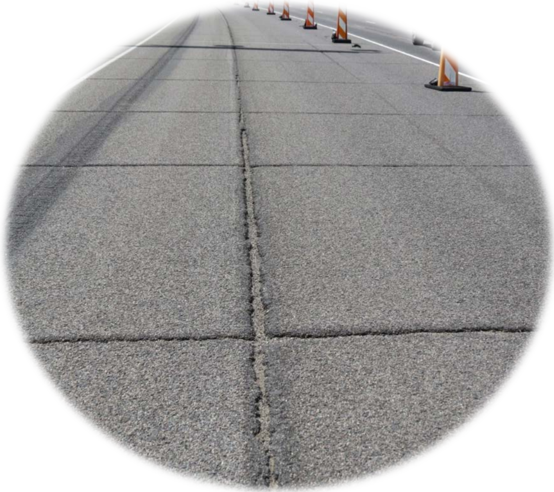
Cracking (Unacceptable)
