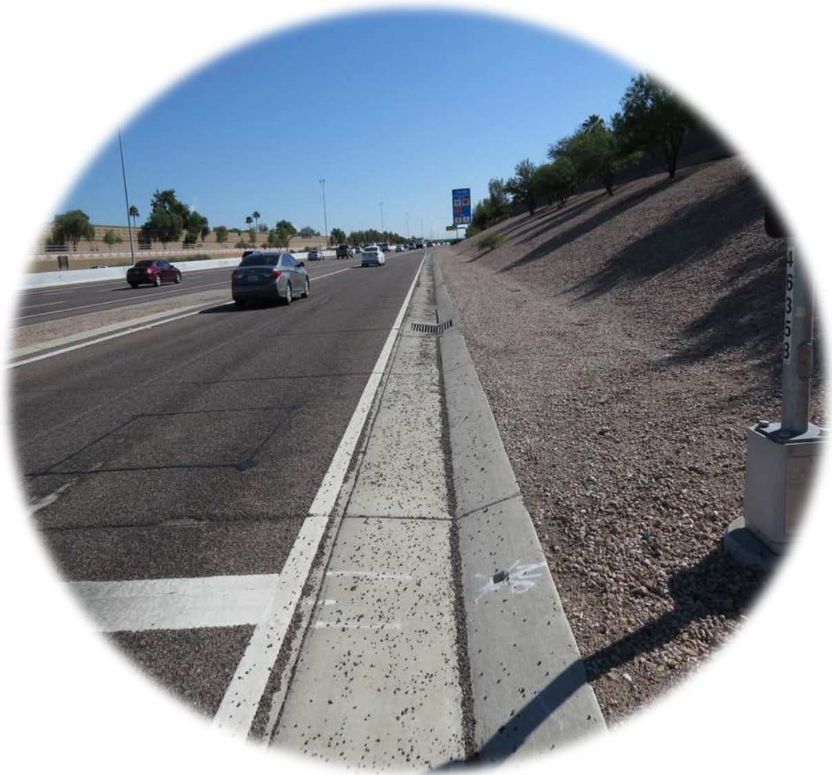
Material accumulation outside of travel lanes (Unacceptable)
