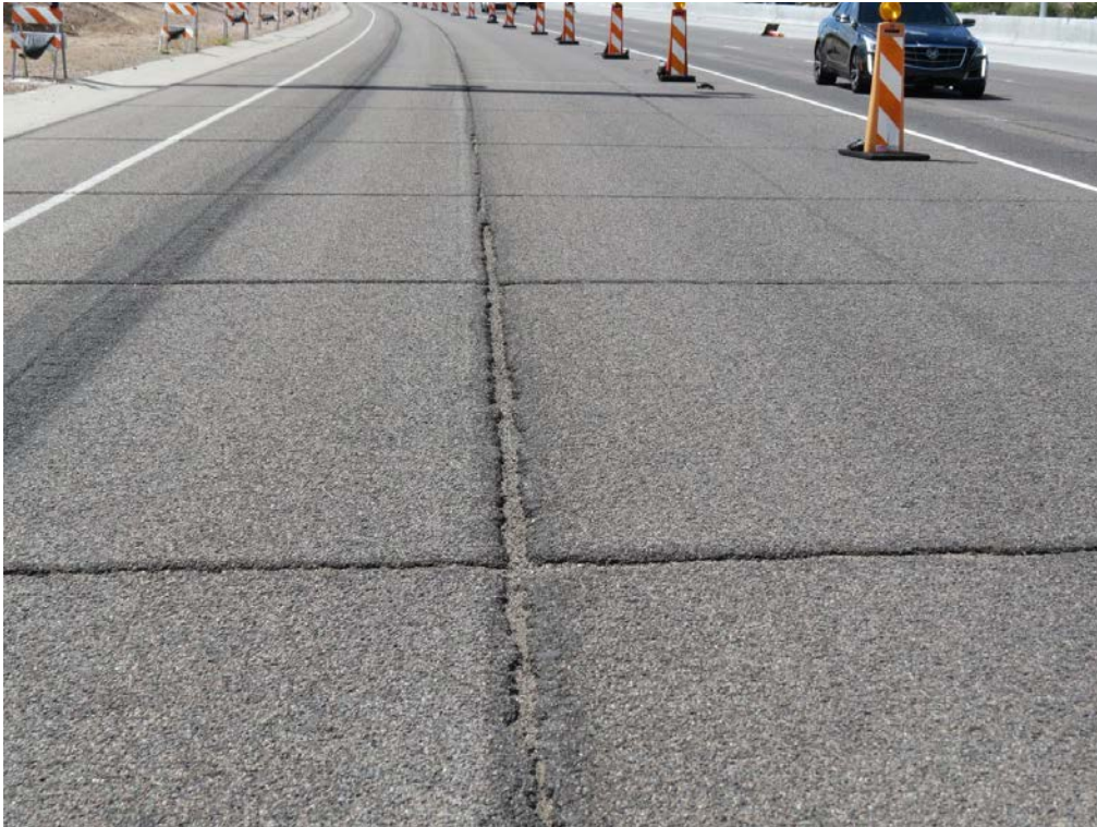
Cracking (Unacceptable)
