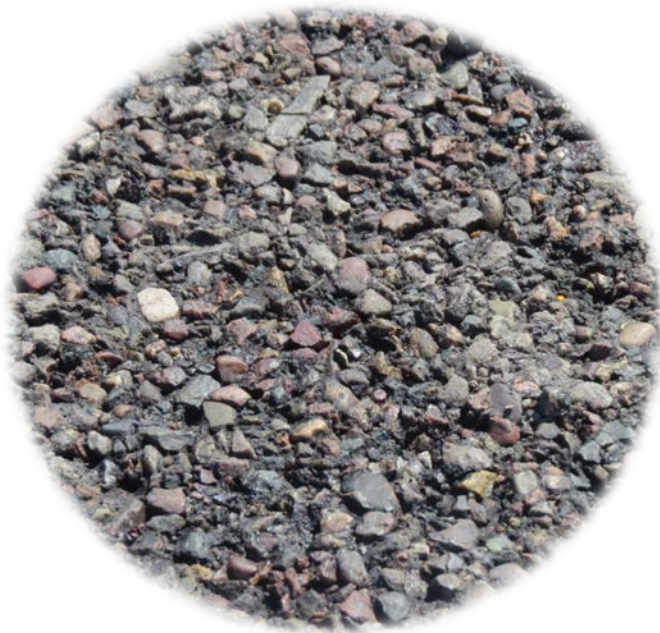
AR-ACFC Rating Unacceptable Pavement
