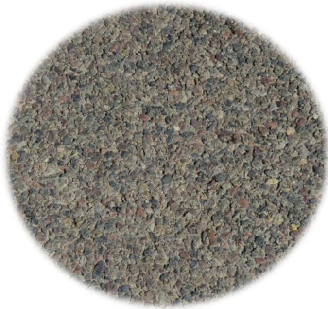
AR-ACFC Rating Good Pavement
