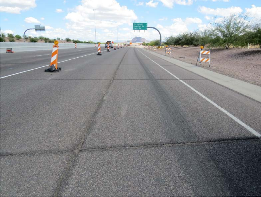
Cracking (Unacceptable)
