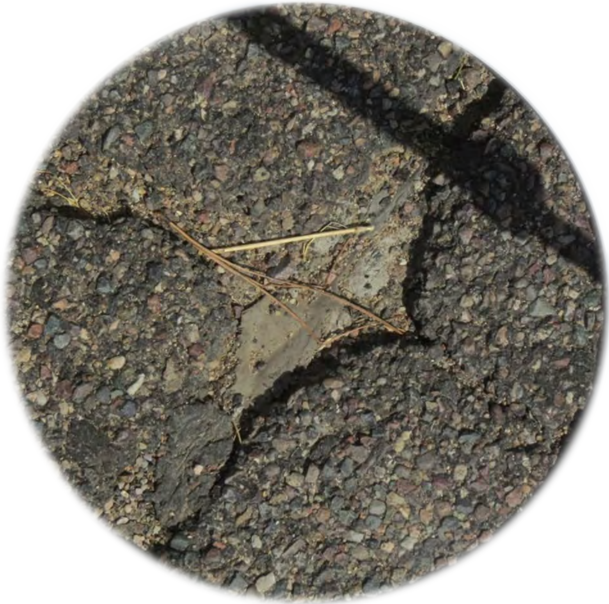
Delamination (Unacceptable)
