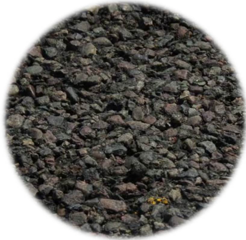
AR-ACFC Rating Unacceptable Pavement
