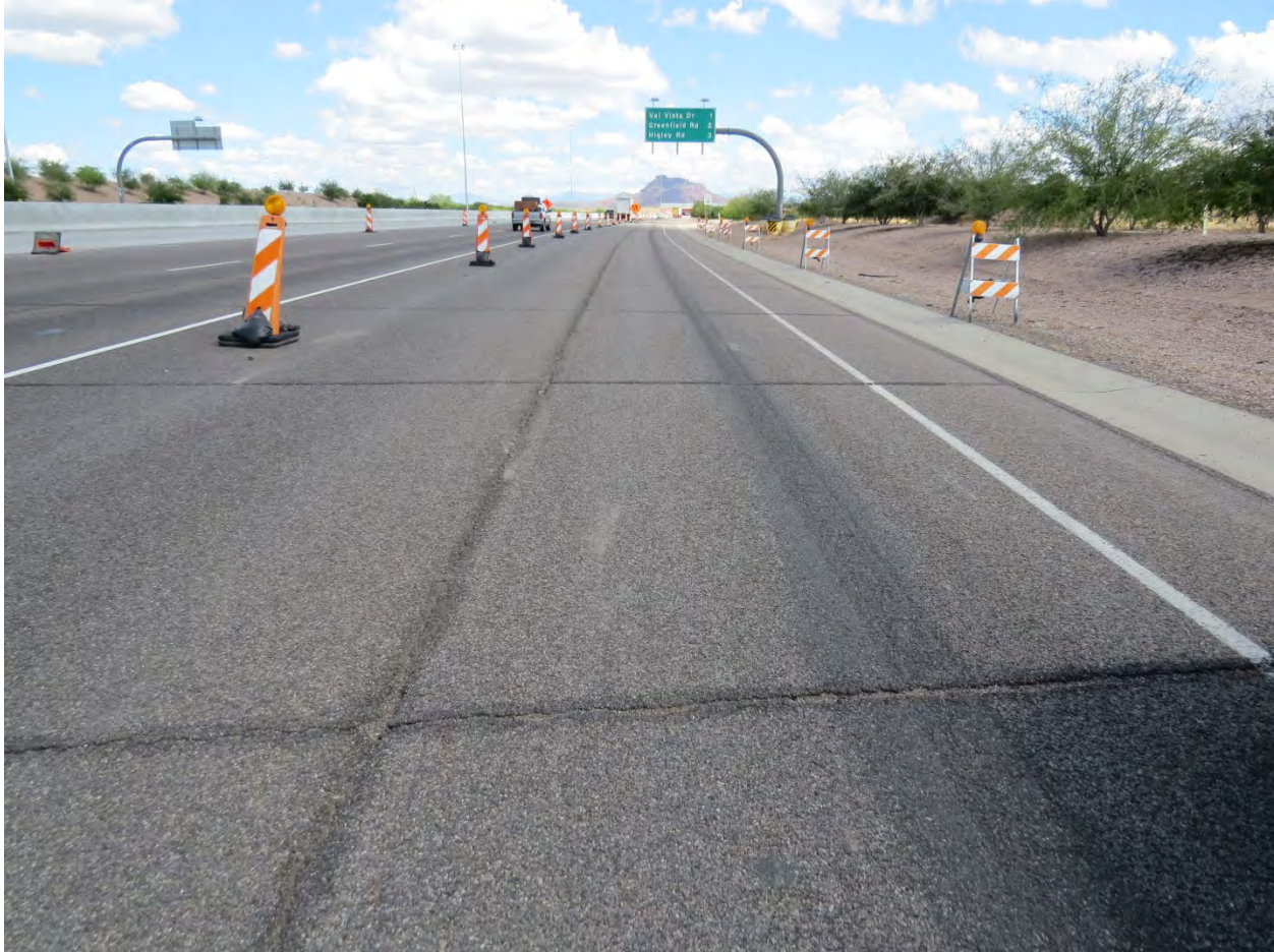
Cracking (Unacceptable)
