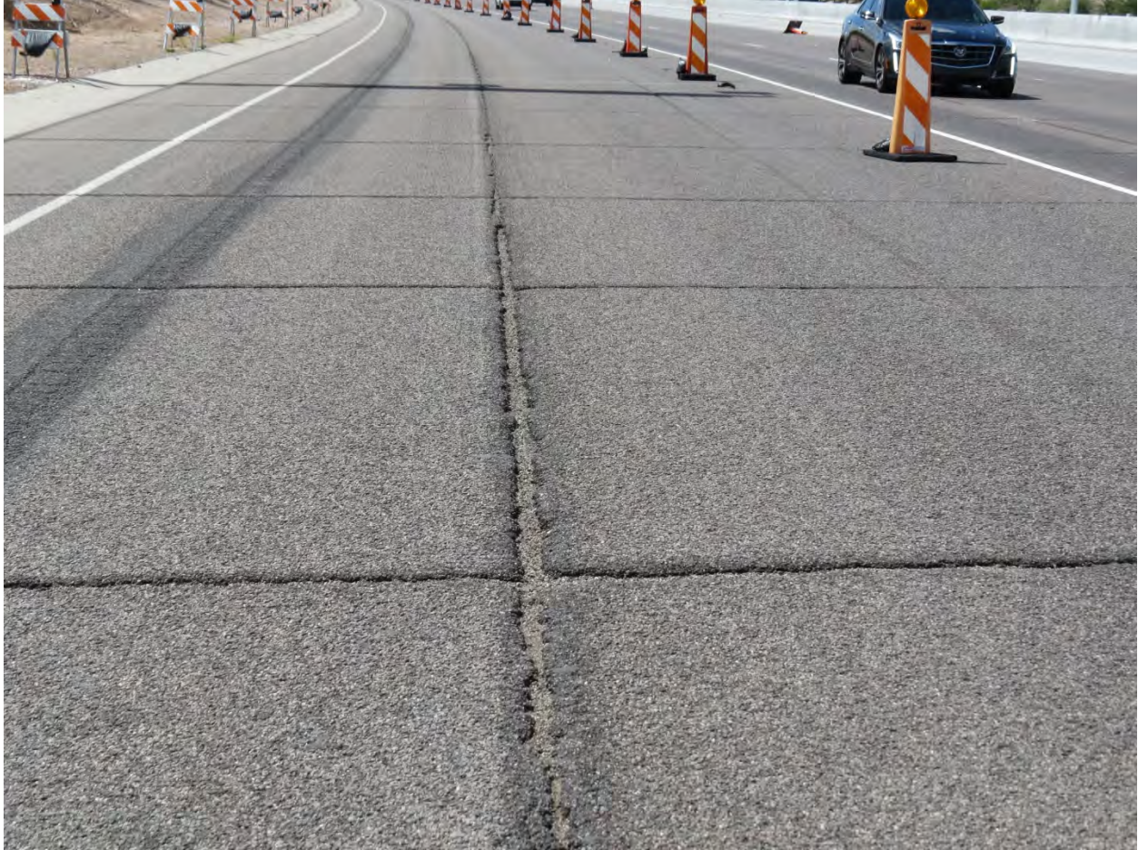
Cracking (Unacceptable)
