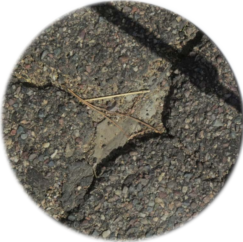
Delamination (Unacceptable)
