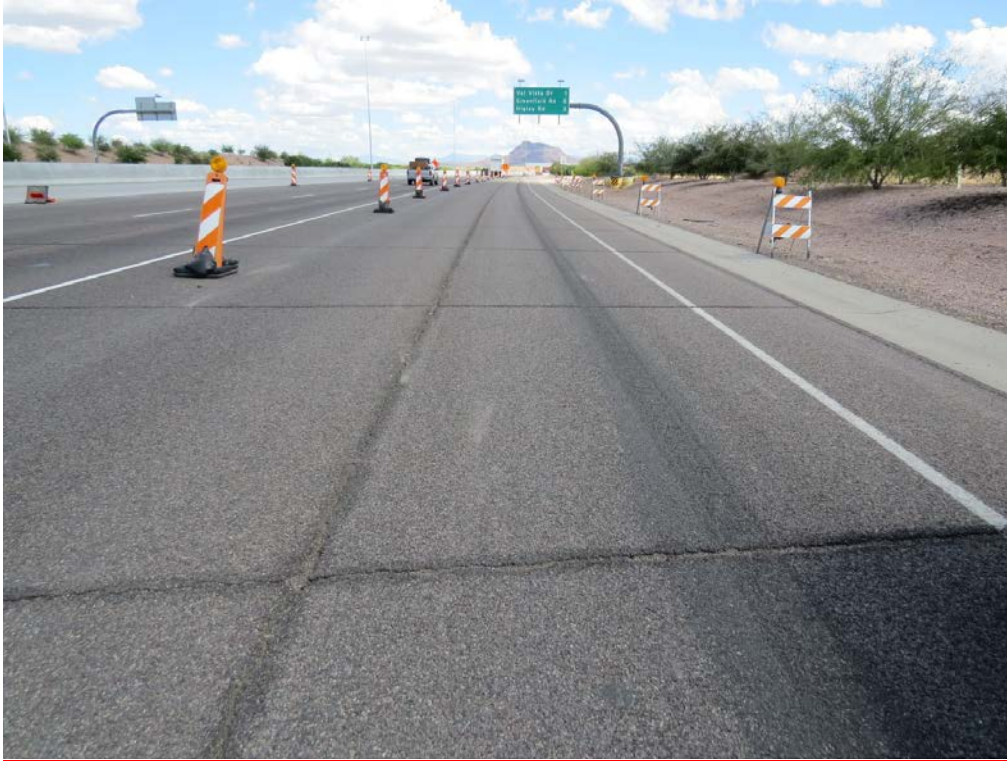
Cracking (Unacceptable)
