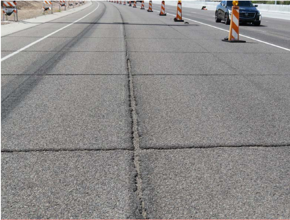
Cracking (Unacceptable)
