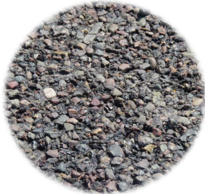
AR-ACFC Rating Unacceptable Pavement
