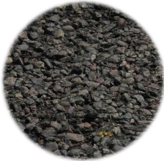
AR-ACFC Rating Unacceptable Pavement
