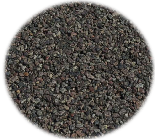
AR-ACFC Rating Unacceptable Pavement
