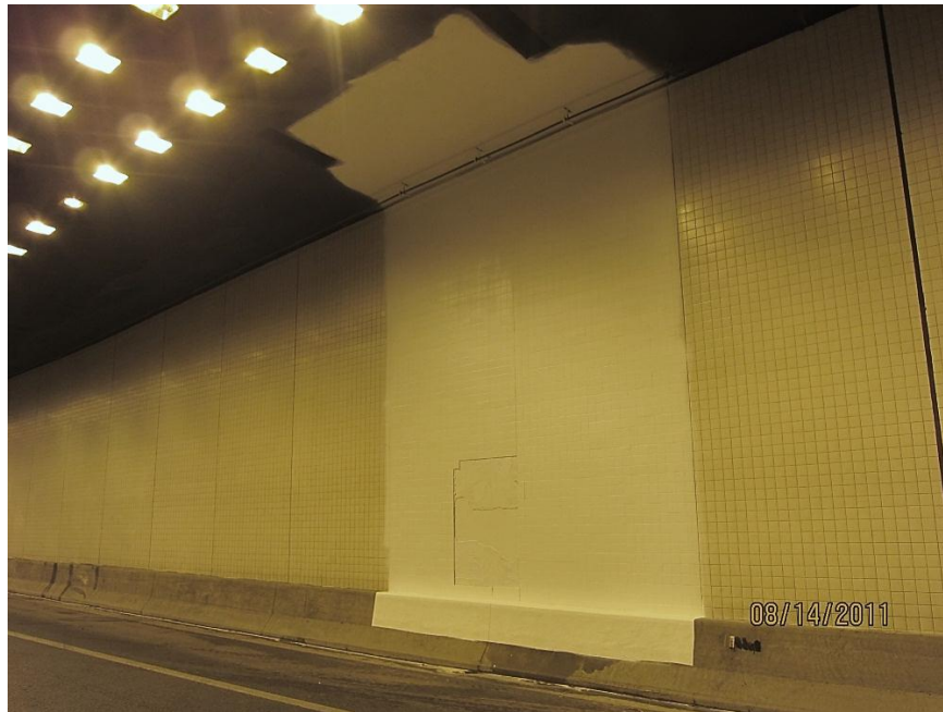
Photo of the Test Area inside the eastbound threshold where the white coating has been applied to the ceiling (See Attachment #3)
