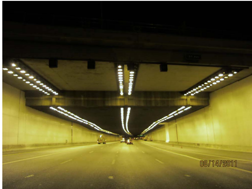
Vertical “Bulkheads” inside the eastbound threshold that should be treated with a high-reflectance white coating
