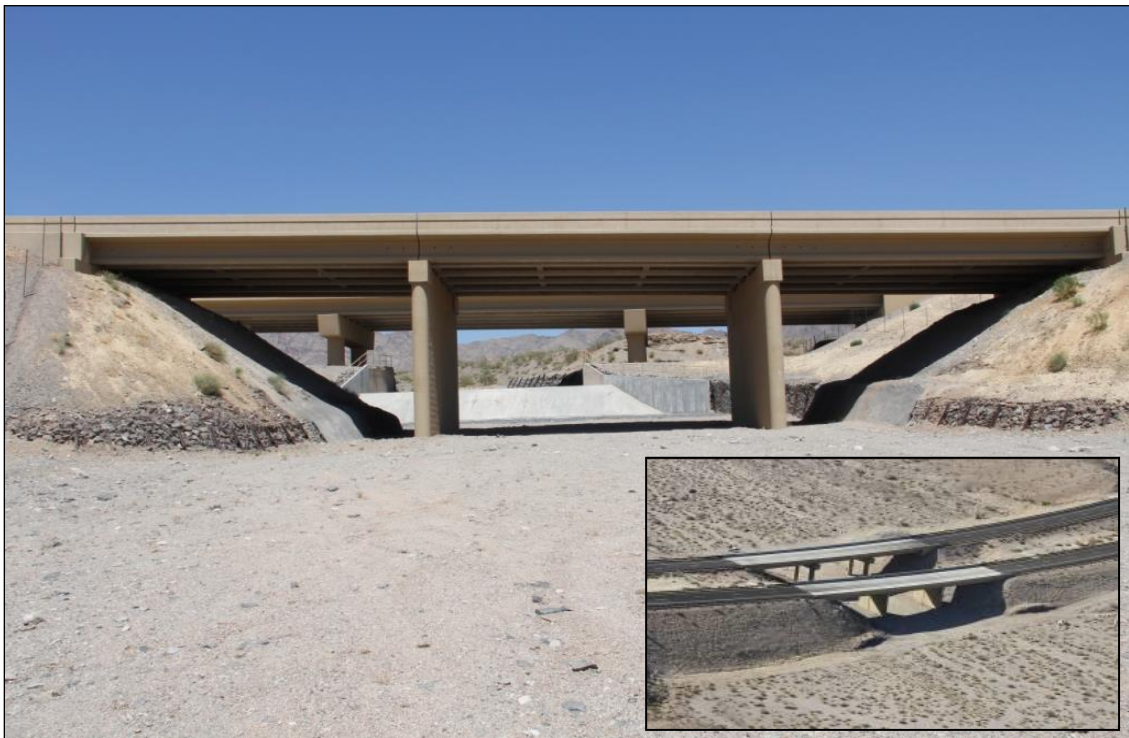
Figure 7. Ground View with Aerial Inset of White Rock Canyon Bridge at MP 4.0 (top) and Devils Wash Bridge at MP 8.0 (bottom) along U.S. 93 near Hoover Dam
