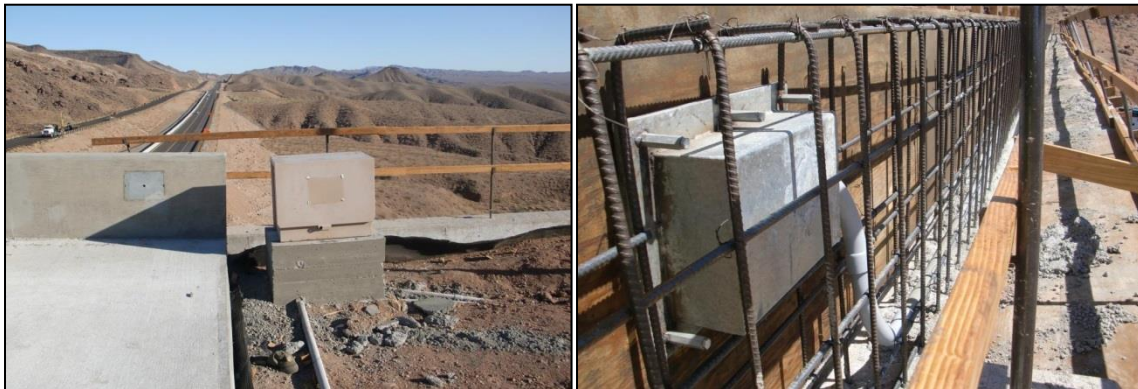
Figure 15. During Wildlife Overpass Construction, State-of-the-Art Video Surveillance Systems Were Incorporated into the Overpass Infrastructure.
