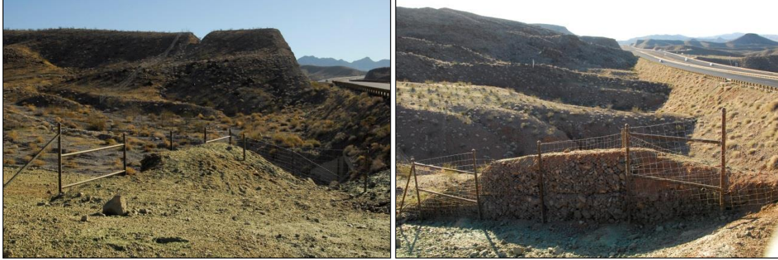
Figure 20. Two Examples of U.S. 93 Escape Ramps with the gradual ramp inside the U.S. 93 ROW sloping up to a designed fence low point (left) and the six-foot drop on the non-ROW side (right). U.S. 93 escape ramps allow animals an opportunity to exit the ROW while minimizing the opportunity to access the ROW.
