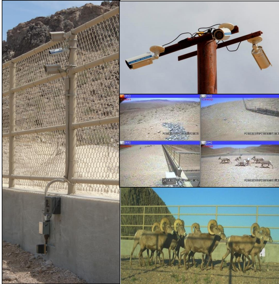
Figure 16. Overpass Surveillance System Components and Resulting Imagery
