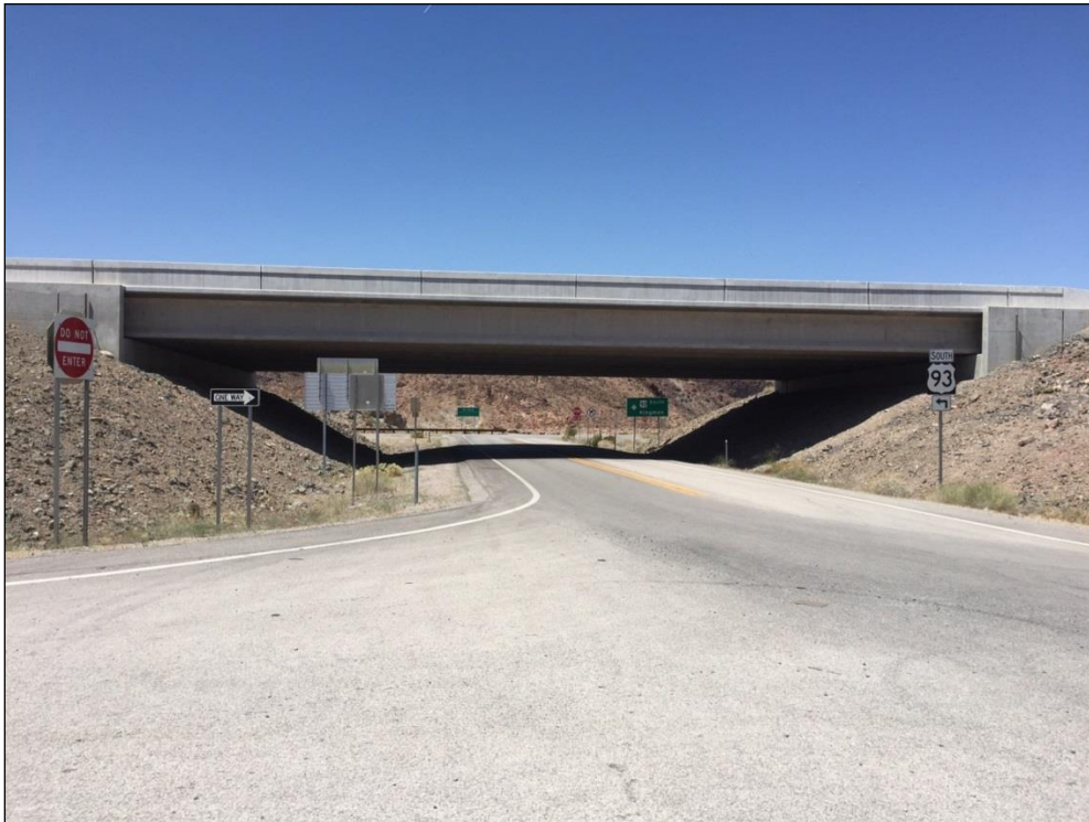
Figure 5. Sugarloaf Mountain Bridge (top) and Kingman Wash Traffic Interchange Bridge (bottom), Both Built as Part of Hoover Dam Bypass Project.
