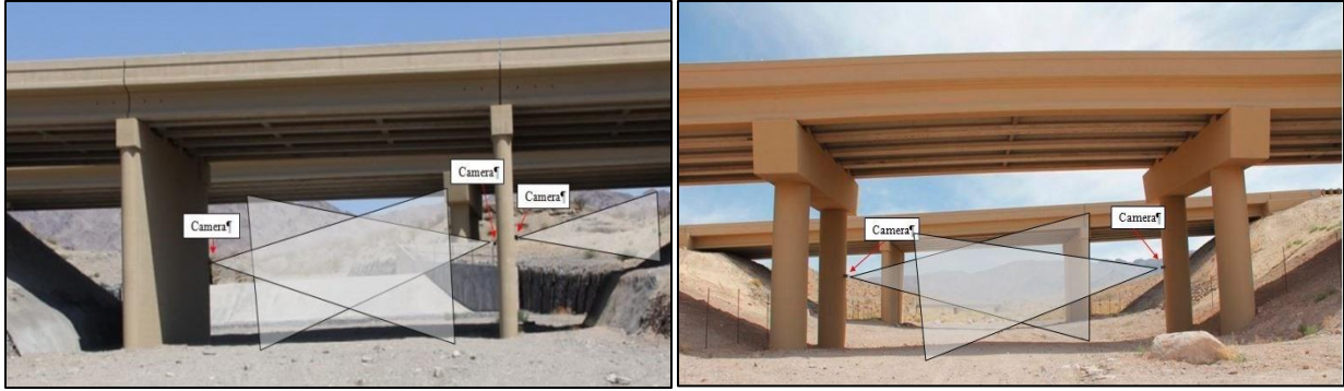
Figure 17. Devils Wash (left) and White Rock Canyon (right) Bridges with Cameras Below. Still camera placement denoted by red arrows, camera orientation by semi-transparent triangles.
