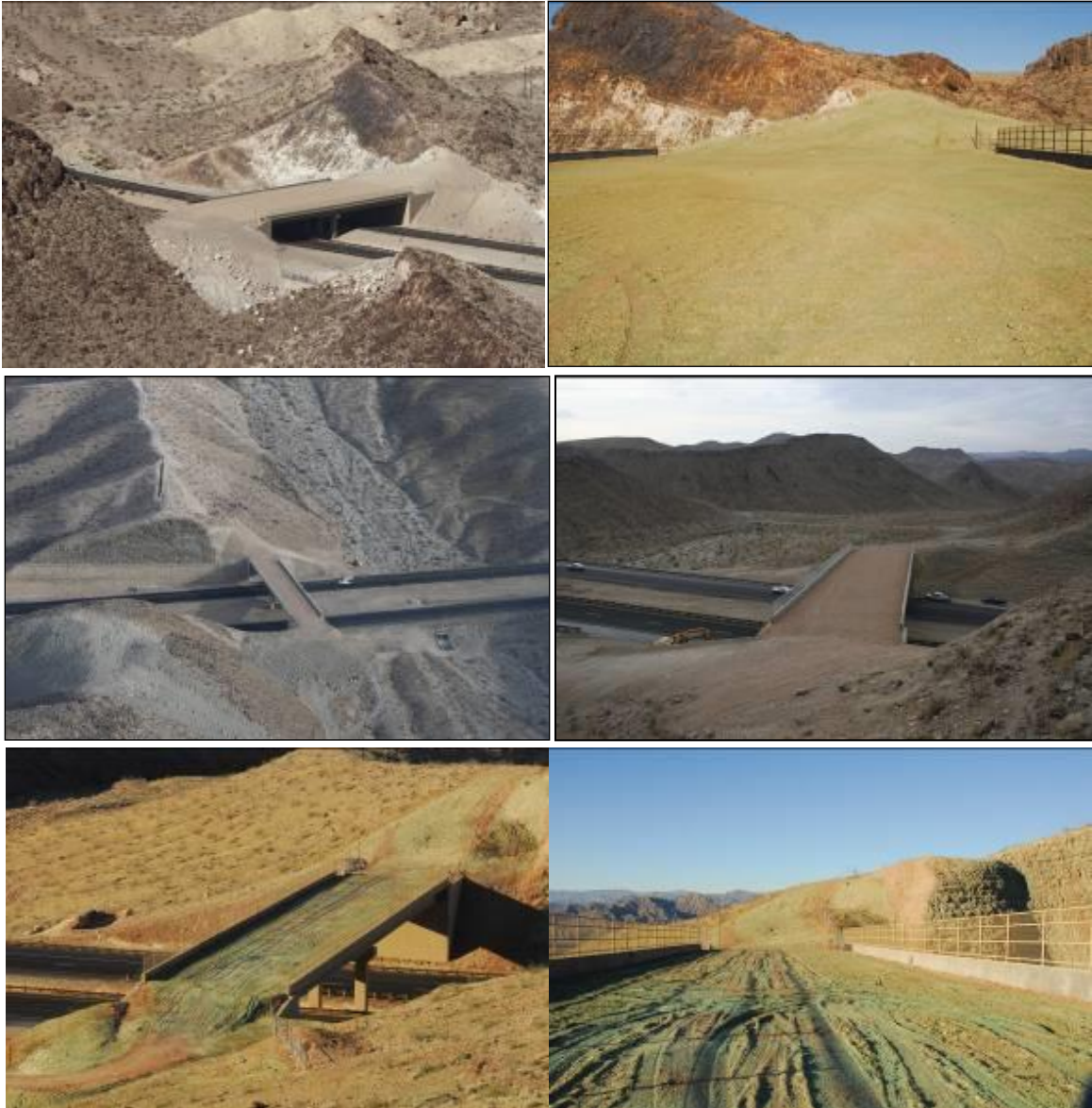
Figure 6. Aerial Views (left column) and Ground Views (right column) of Wildlife Overpasses Built along U.S. 93 at MP 3.3 (top), MP 5.2 (middle), and MP 12.2 (bottom)
