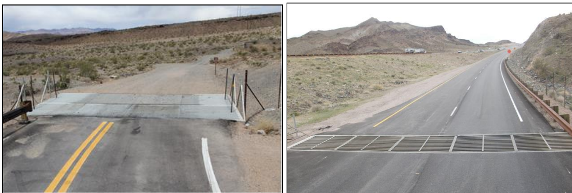
Figure 21. Example of a Double-Wide (left) and Single-Wide (right) Cattle Guard on U.S. 93
