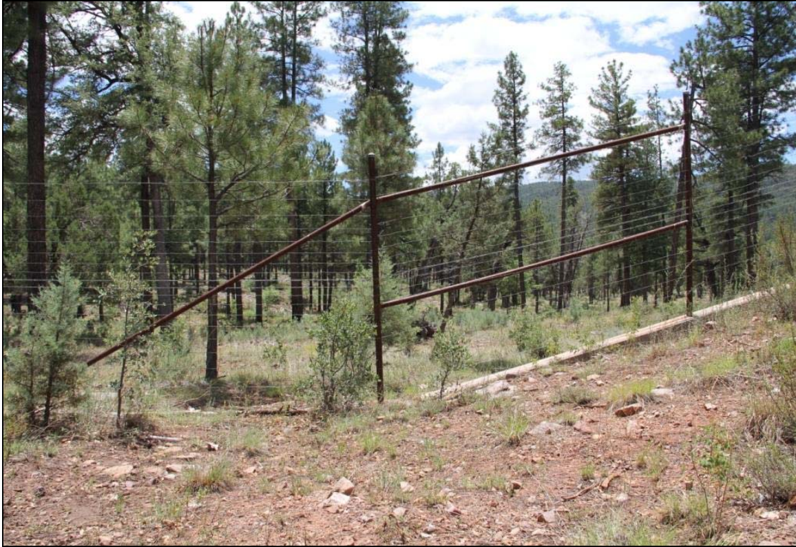
Figure 25. Example of Standard Woven Wire Ungulate-Proof Fence Recommended for Interstate 17
