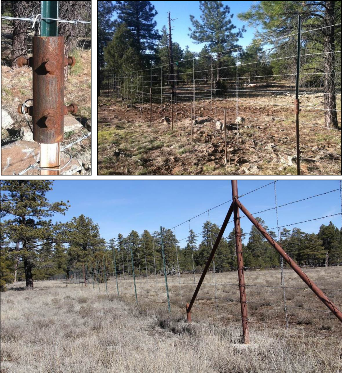
Figure 8. Heightened Fencing along the Study Area: Metal Couplers Attached Extensions to Existing T-Posts (Top Panel); New 8-Ft-High Fencing Replaced Fencing that Was Too Degraded to Heighten (Bottom Panel)
