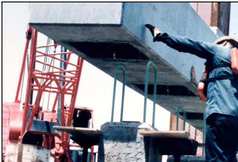
Figure 17. Precast Cap on Red Fish Bay and Morris and Cummings Cut Bridge. (Wolf 2005.)
