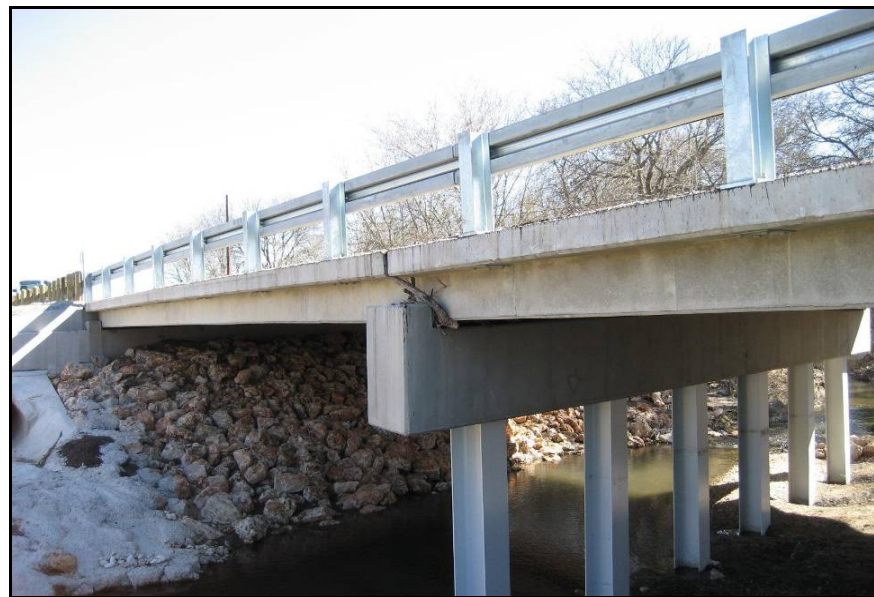
Figure 31. Completed Cottonwood Creek Bridge. (Marin 2008.)
