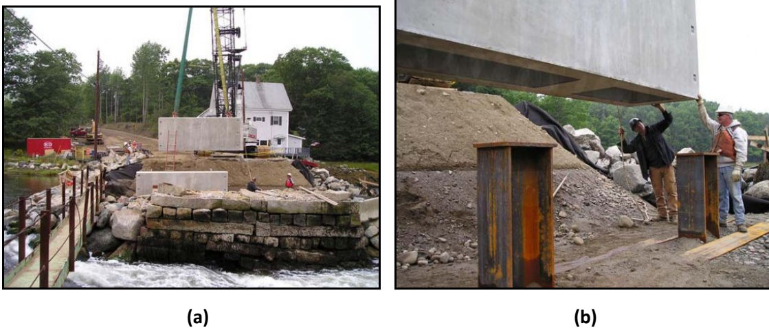
Figure 10. Construction of the All-Prefabricated David Narrows Bridge. (PCINE 2006.)
