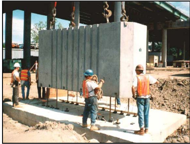
(b) Pier Footing Connection
