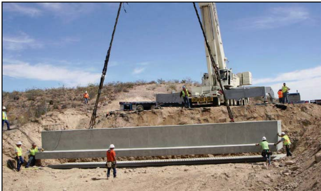
Figure 4. Precast Concrete Abutment at Marble Wash Bridge, I-40. (Blanchard et al. 2009.)
