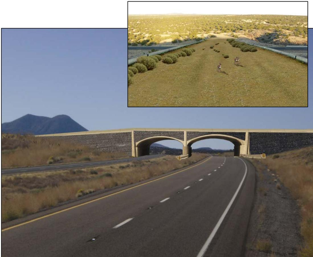
*Figure 17.* Rendering of a CON/SPAN<sup>®</sup> pre-cast concrete arch application for a wildlife overpass at MP 440.9 along US 89. The bottom rendering depicts separate 32-ft spans (21 ft high) over each set of lanes, looking south, and the inset depicts the top of the overpass, looking east (note: fencing would need to be erected atop the walls).
