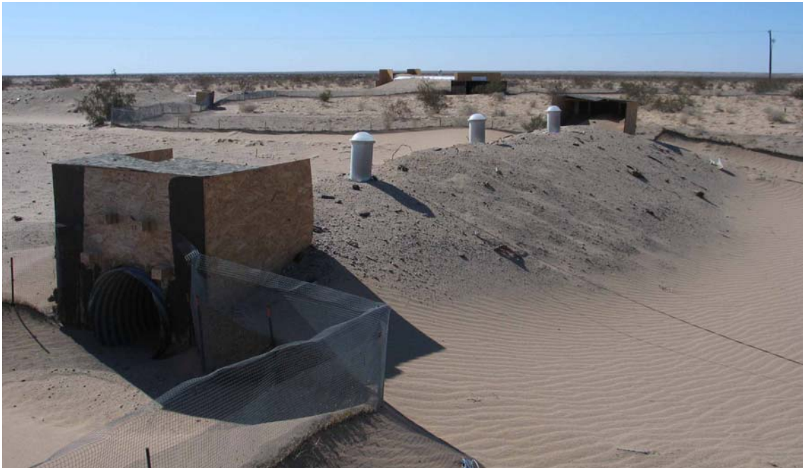
Figure 5. Skylights positioned on a 24-in diameter culvert.
