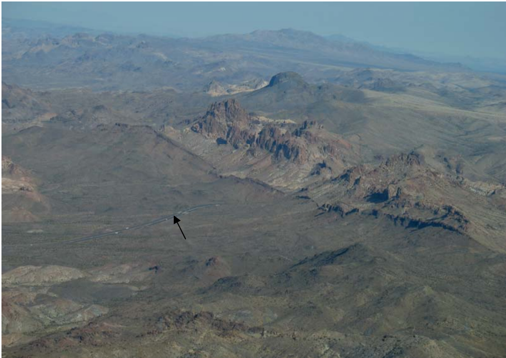
Figure 3. The Hole wildlife underpass (MP 10.8) on State Route 68 in northwestern Arizona, 2005-2007.
