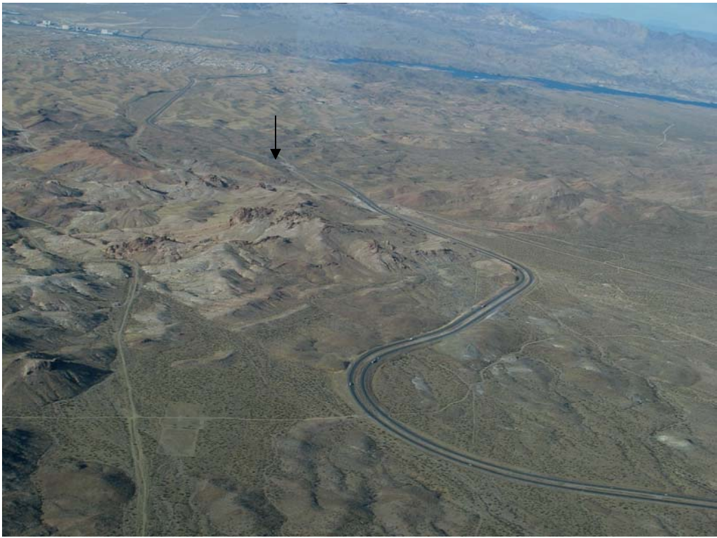
Figure 4. Arabian Mine wildlife underpass (MP 7.8) on State Route 68 in northwestern Arizona, 2005-2007.
