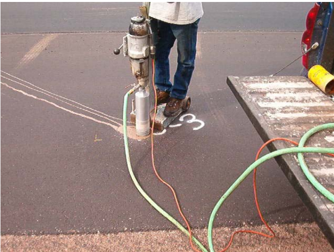
Figure N.26 – Coring at Site 9
