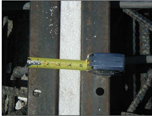
Photograph 7: Joint measurement prior to setting
