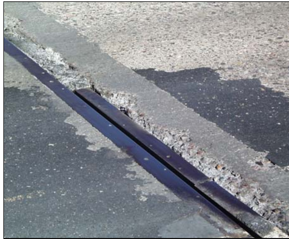
Photograph 8: Failed concrete header and angle armor
