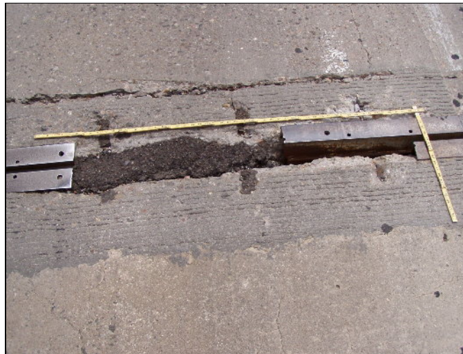
Photograph 12: Repair of bridge deck joint due to snowplow
