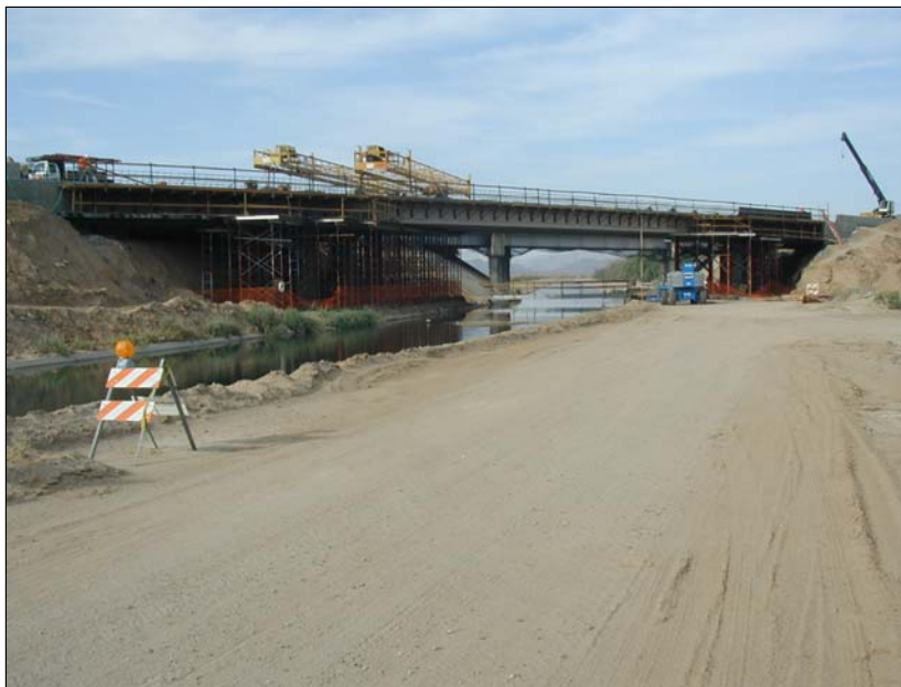
Photograph 1: Bridge replacement under construction
