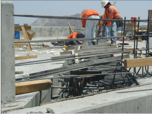
Photograph 9: Deck joint under construction
