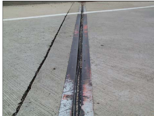
Photograph 4: Adhesion failure of compression seal
