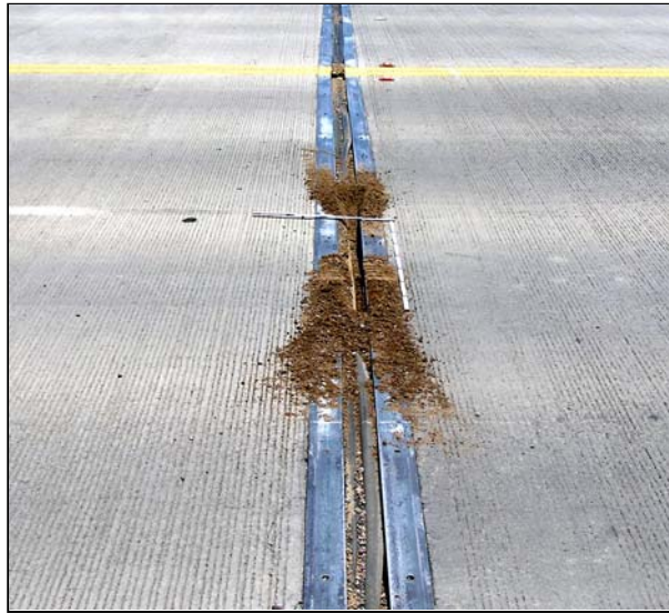
Photograph 5: Debris compacted compression seal
