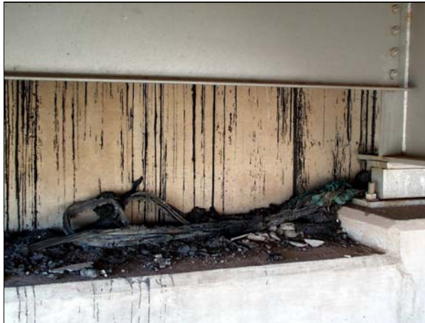
Photograph 3: Failed compression seal
