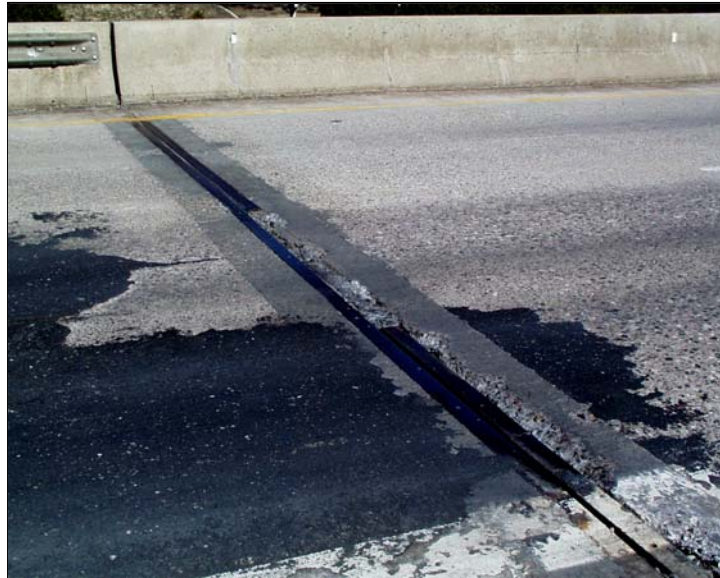
Photograph 11: Bridge deck joint damaged by snowplow
