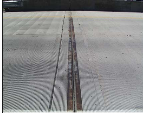
Photograph 2: In-service compression joint
