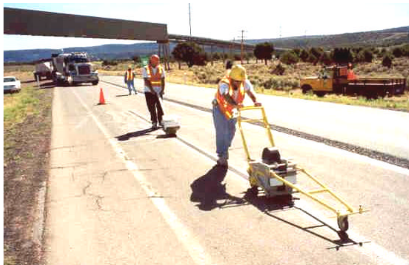
Figure 6: Test Installation of 3M Tape at Black Mesa
