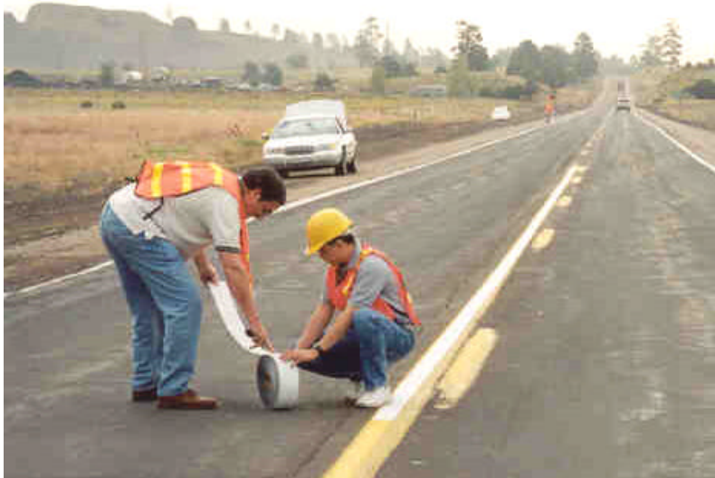
Figure 10: Temporary 3M Tape on Old Route 66 for Commissioning System
