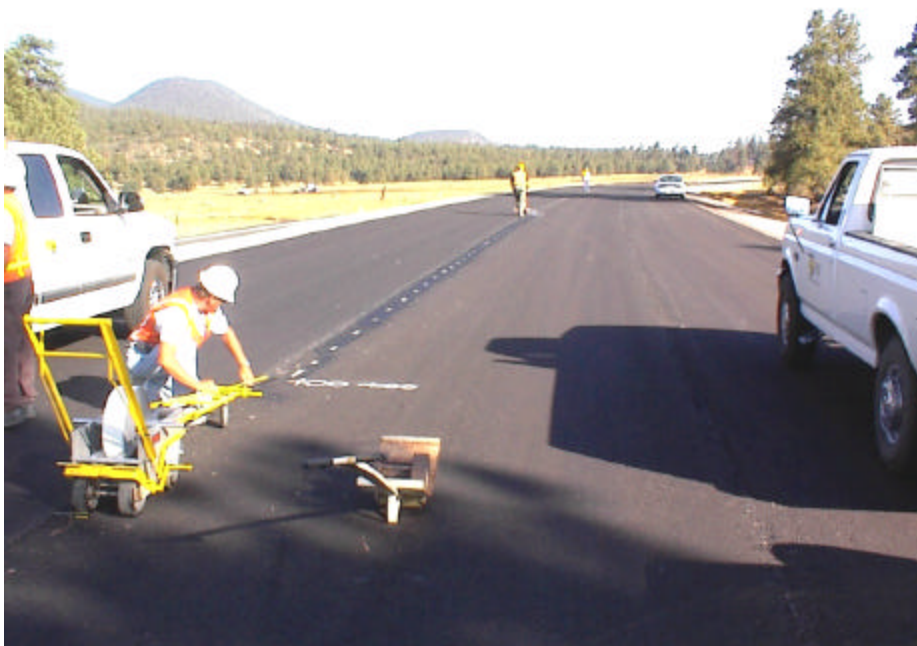
Figure 7: Tape Layout and Adhesive Placement - US 89
