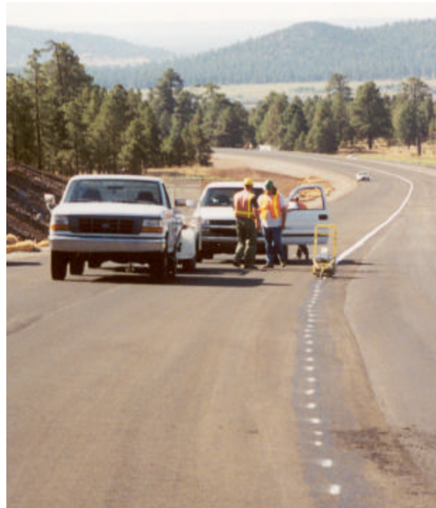
Figure 8: Installation of 3M Tape on US 89
