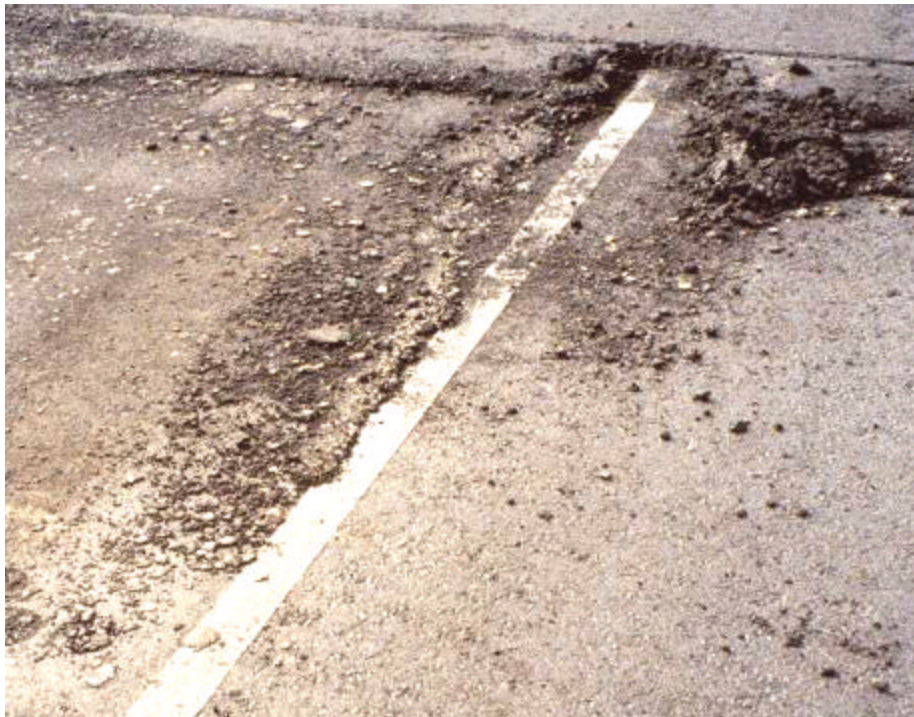
Figure 4: Underlay Installation of 3M Tape
