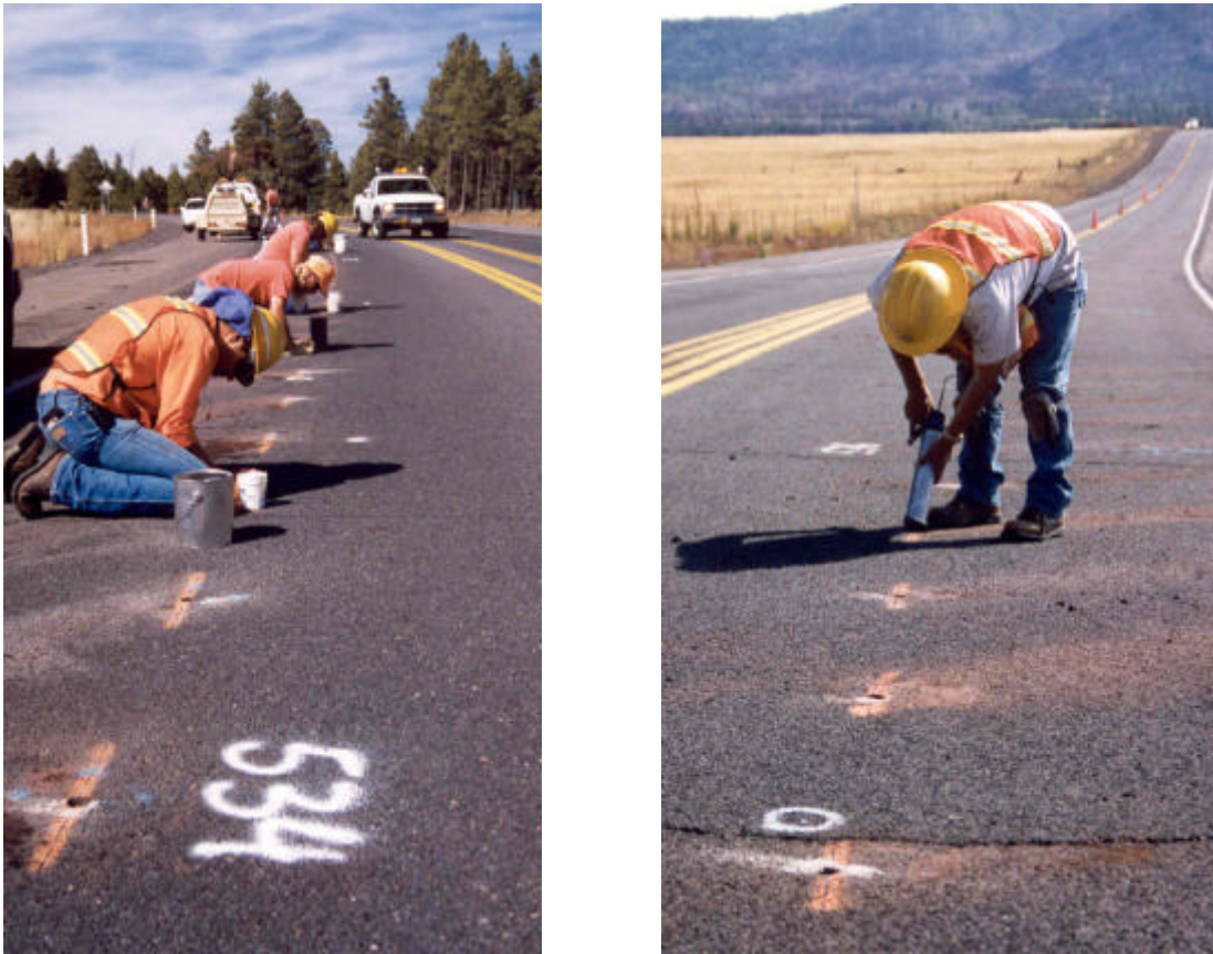
Figure 26: Setting and Sealing the PATH Magnets
