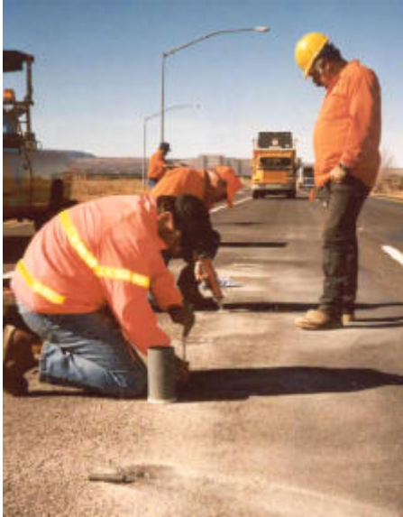
Figure 14: Installing and Sealing Test Magnets on I-40
