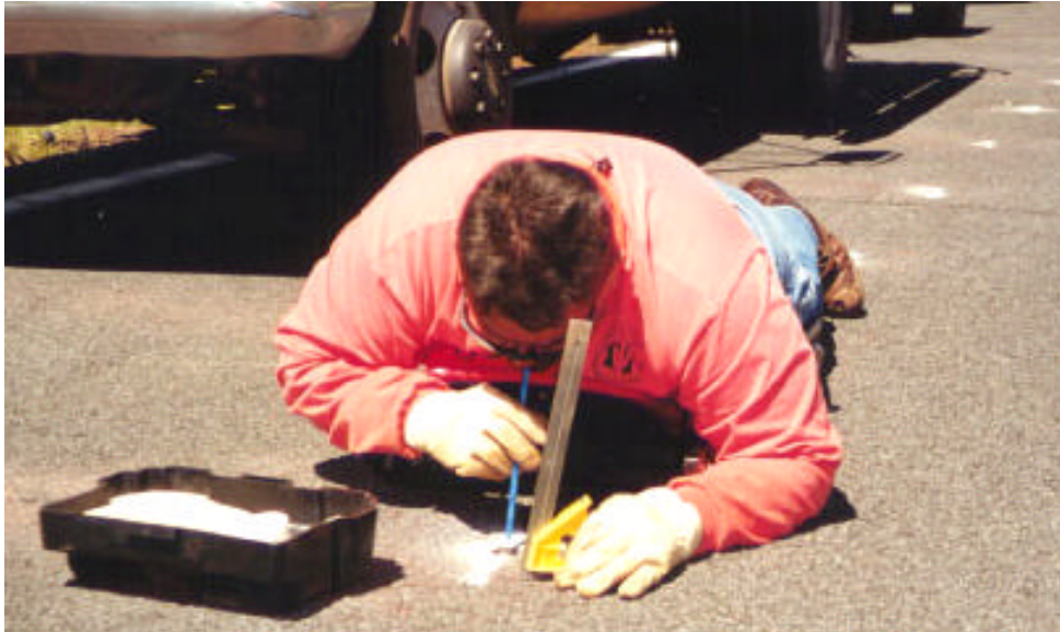
Figure 28: Installing Magnets
