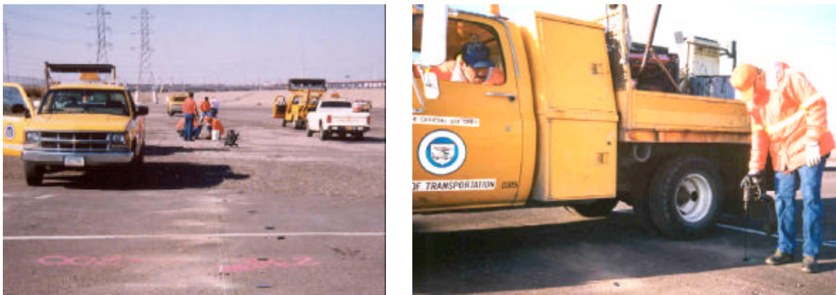
Figure 5: Placing and Sealing Magnets with Hot Adhesive at ASU Stadium Demo Site
