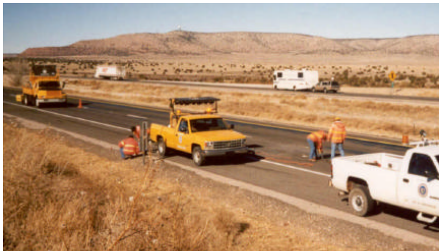
Figure 13: Test Magnet Installation at Seligman (I-40 MP 121.0)
