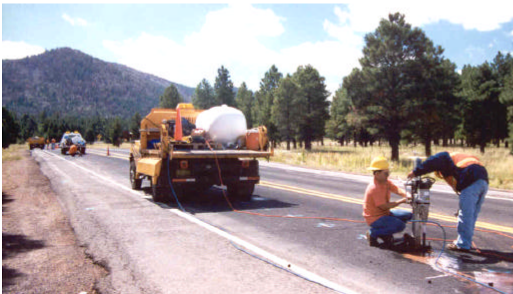
Figure 25: Four Two-man Crews on the Drill Line
