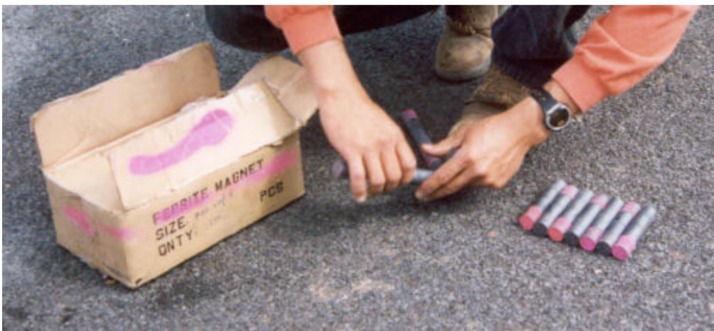
Figure 10: California PATH Discrete Magnetic Markers
