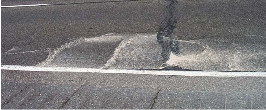
Figure 77. A Fatigued Area with Pumping on Section 040661 (August 2000).
