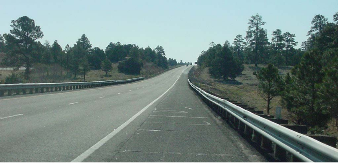
Figure 6. Section 040662 Constructed Over Fill.
