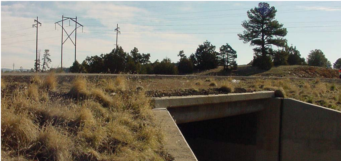
Figure 4. Box Culvert in Section 040660.
