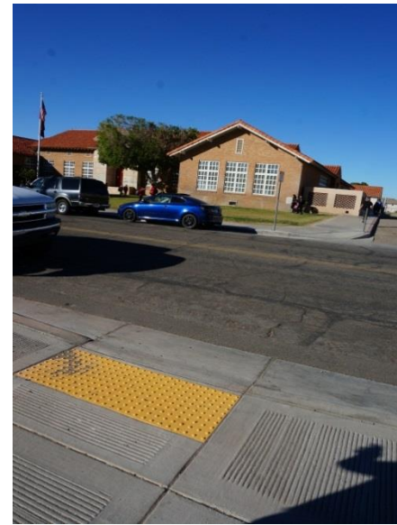
Existing accessible ramp on 5th Street in front of school
