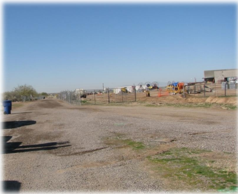
View of Park Street, looking west. Construction of Multipurpose Center seen at right
