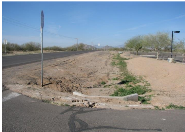
Sidewalk placement on Santan Road will need to consider existing drainage culvert locations. This is a view of Santan Road, looking west, at the District 4 Service Center.
