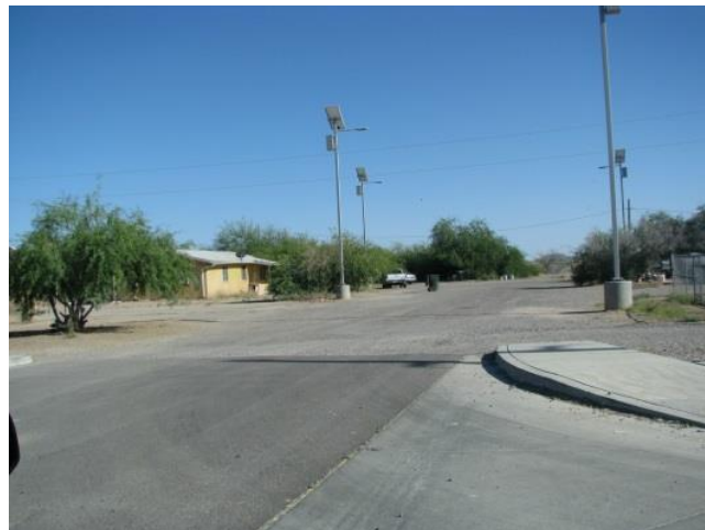
Eagle Court, looking south from Casa Blanca Road
