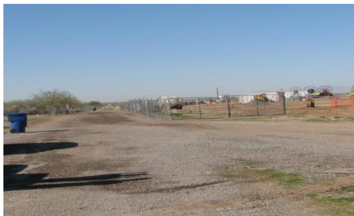
Park Street looking west, construction of Multipurpose Center at right of photo
