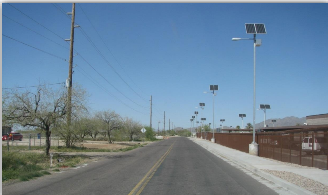
New sidewalk and street lighting on Cholla Road, adjacent to the Head Start.
