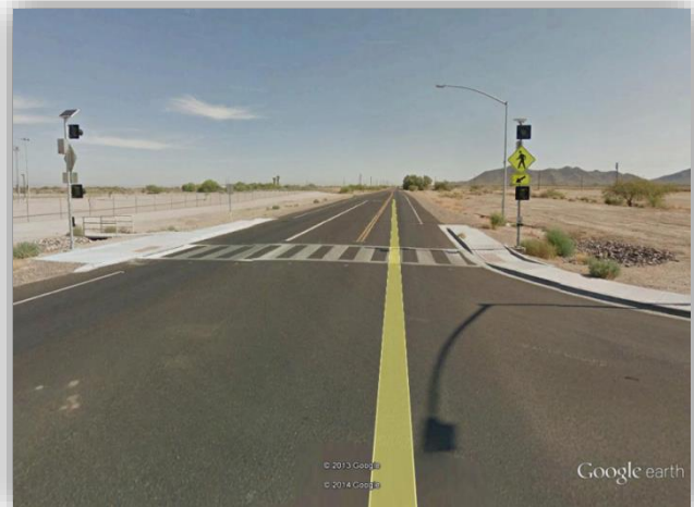
Crosswalk at 51 st Avenue/Tashquinth Drive
