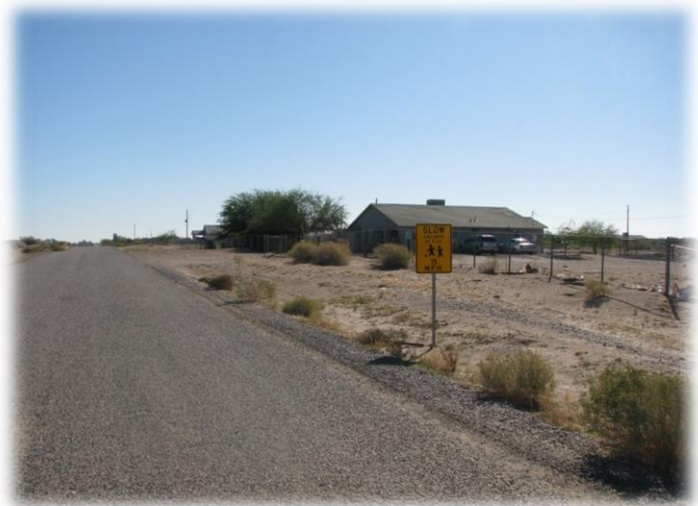
Park Street looking east. Note the lack of walking or biking areas adjacent to the road.
